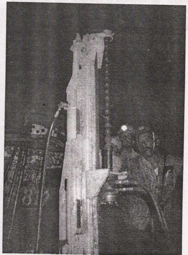
drilling in progress
